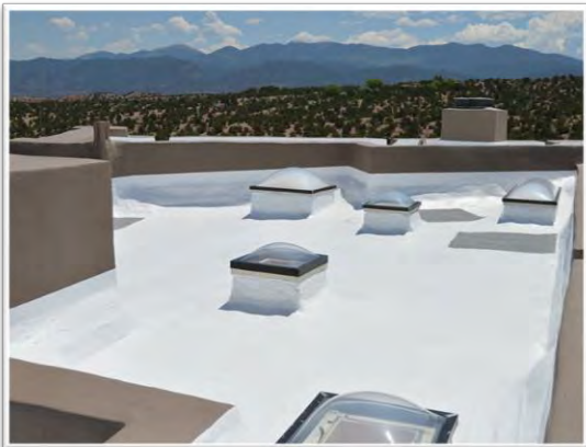
Elastomeric roof coating
